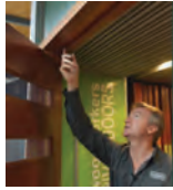
adjusting and weather sealing a pivot door
