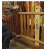
how to measure & install balustrade
