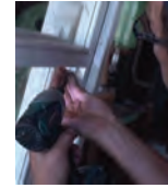
removing & refitting spiral balances
